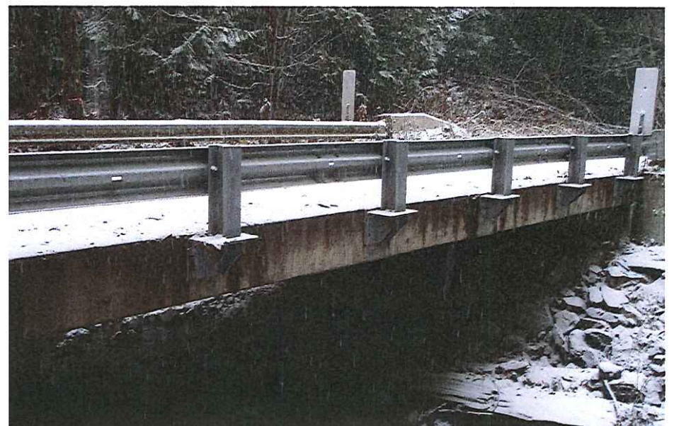
CK-2046 Crossing Downstream
