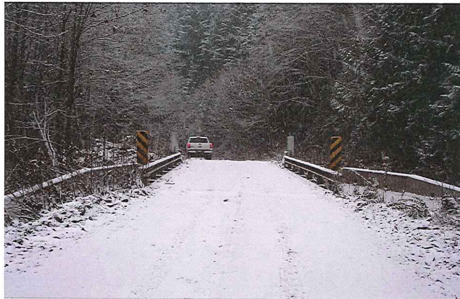
CK-2046 Approach Right Bank
