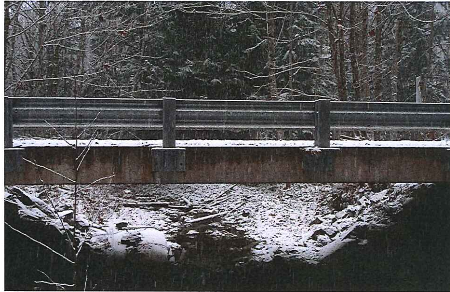
CK-2046 Crossing Upstream
