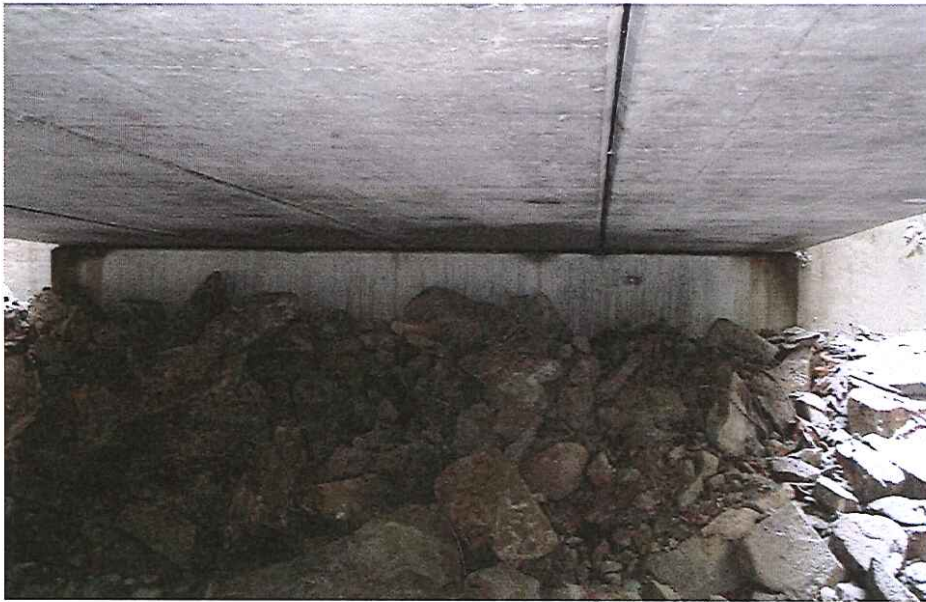
CK-2046 Abutment Right Bank
